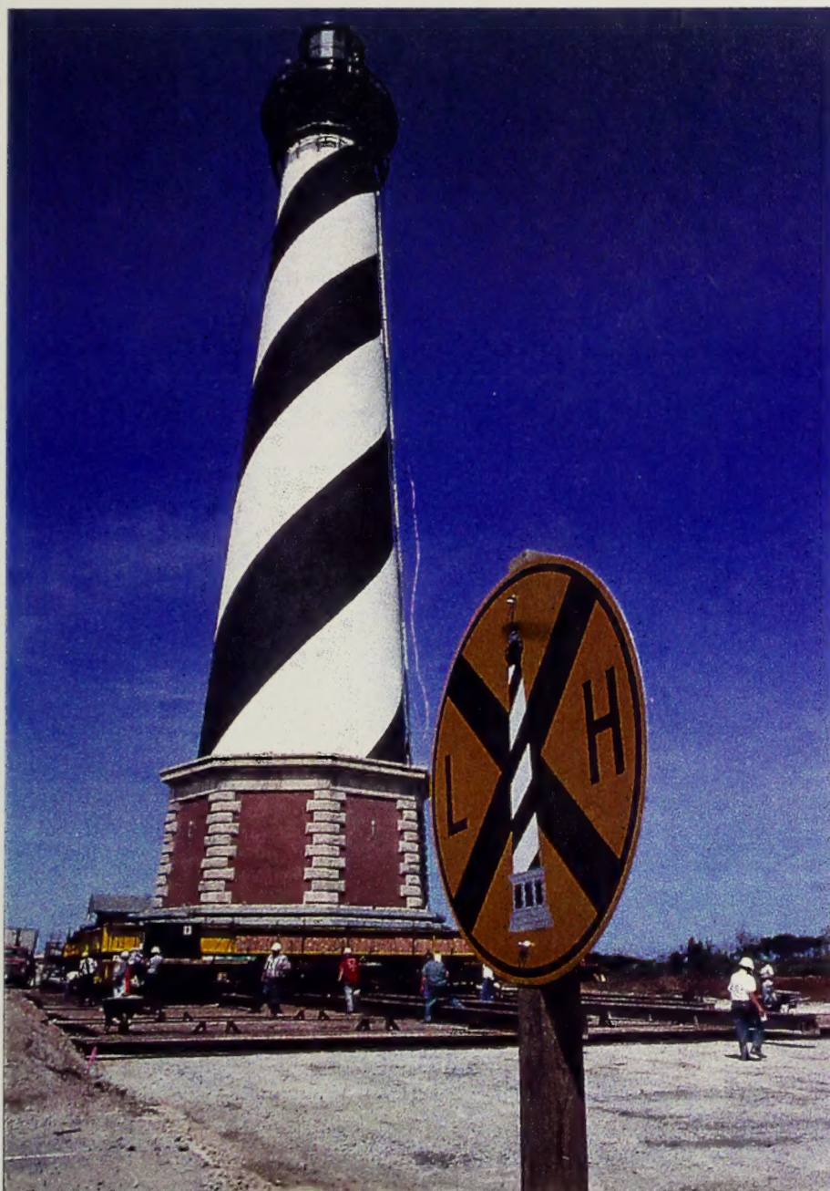
LIGHTHOUSE PROJECT WINS AWARD: The American Society of Civil Engineers named the Cape Hatteras Light Station Relocation Project as the nation's outstanding civil engineering achievement.
