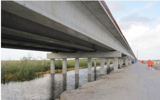
The Tamiami Trail Next Steps Project is enhancing the connectivity and water flow between the marshes north and south of the Tamiami Trail, while maintaining the vital transportation link between southwest Florida and Miami.
