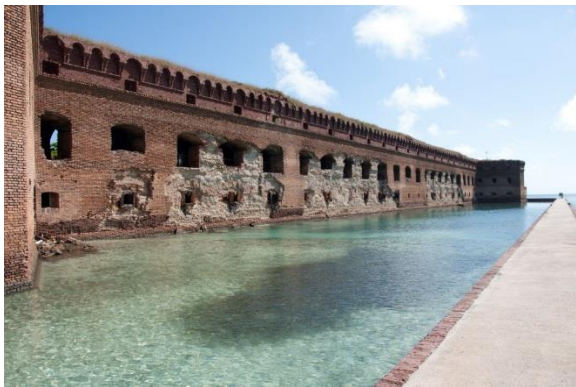
Before and After: Front 3 Comprehensive stabilization of upper and lower embrasures; removal of existing iron Totten shutter assemblies; infill arch reconstruction, replicated shutter component installation; scarp repointing as well as parapet brick replacement and repointing.
