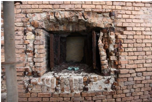
Before and After: Front 3 Lower Level Bastion Embrasure Reconstruction including removal of existing corroded iron Totten shutter assembly components and installation of replicated shutter components along with brick replacement and repointing.
