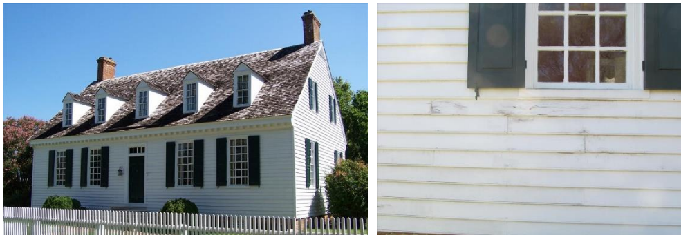
Projects like this at Colonial National Historical Park, to repair and rehabilitate the exterior shell of the Dudley Diggs House. First constructed in 1755 and restored in 1954, the House is along the Main Street—one of the primary visitor pathways—making the structure, and its deteriorating exterior, a significant factor of the visitor experience.
