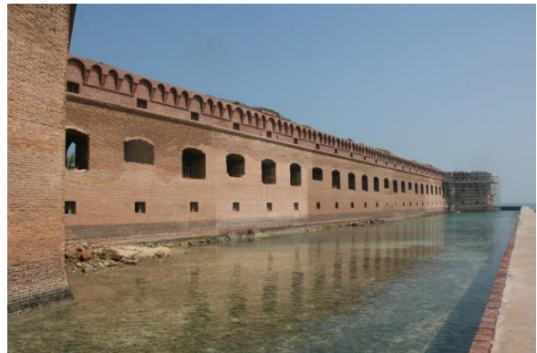
Before and After: Front 3 Comprehensive stabilization of upper and lower embrasures; removal of existing iron Totten shutter assemblies; infill arch reconstruction, replicated shutter component installation; scarp repointing as well as parapet brick replacement and repointing.
