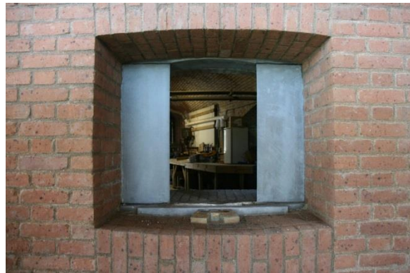
Before and After: Front 3 Lower Level Bastion Embrasure Reconstruction including removal of existing corroded iron Totten shutter assembly components and installation of replicated shutter components along with brick replacement and repointing.
