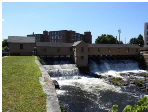
In 2018, the hydropower facilities within Lowell NHP began relicensing proceedings. DOI requested studies include: Resources, Ownership, Boundaries and Land Rights; Water Level and Flow Effects on Historic Resources and Recreation; Vegetation and Aquatic Trash Management; and Historically Significant Water Power Equipment.
