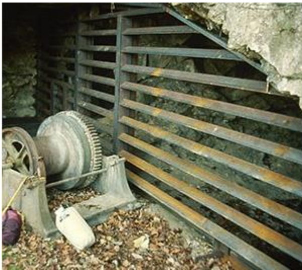
Bat gate mine closure and historic mining equipment at Buffalo National River, Arkansas. NPS photo
