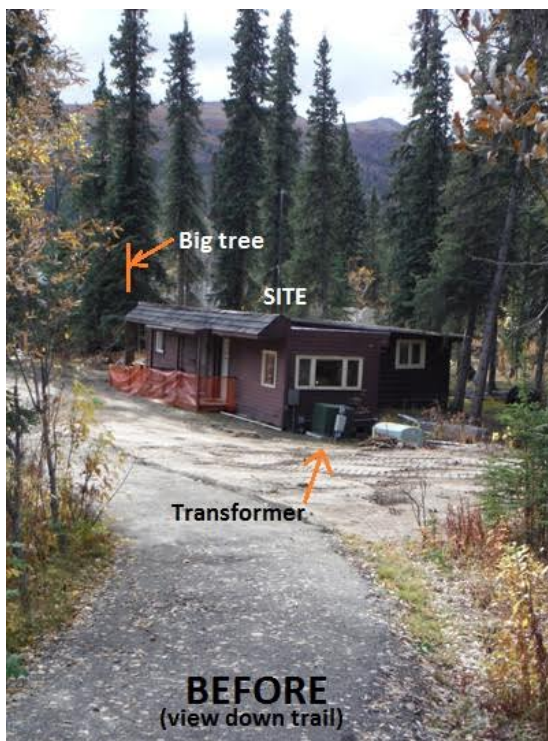
Denali NP&Pres obsolete former dispatch center
