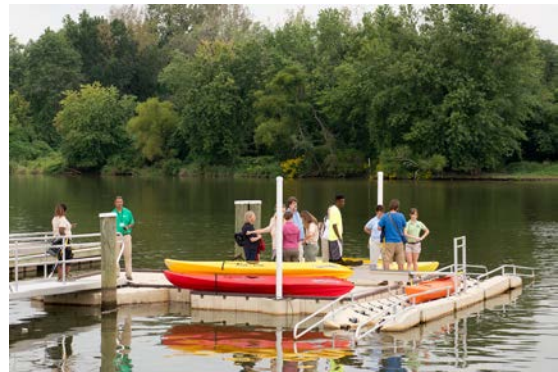
Universally accessible canoe/kayak launch for the Anacostia Water Trail at Bladensburg Waterfront Park, Maryland.
