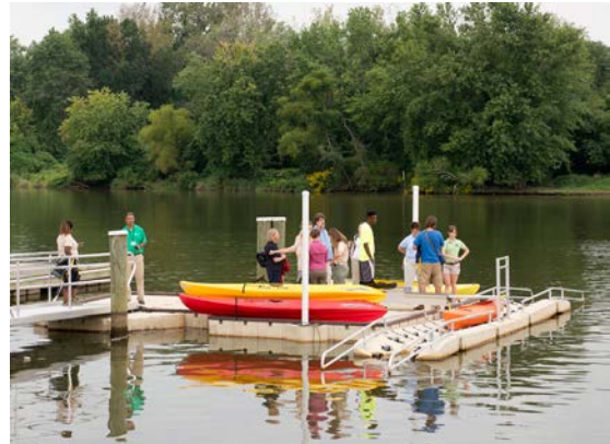
Universally accessible canoe/kayak launch for the Anacostia Water Trail at Bladensburg Waterfront Park, Maryland. NPS photo.
