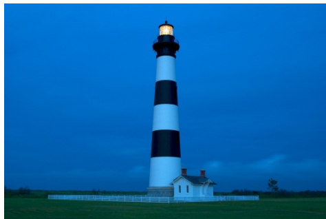
Bodie Island Light Station, Cape Hatteras NS.
