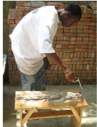
At DC student prepares mortar.
