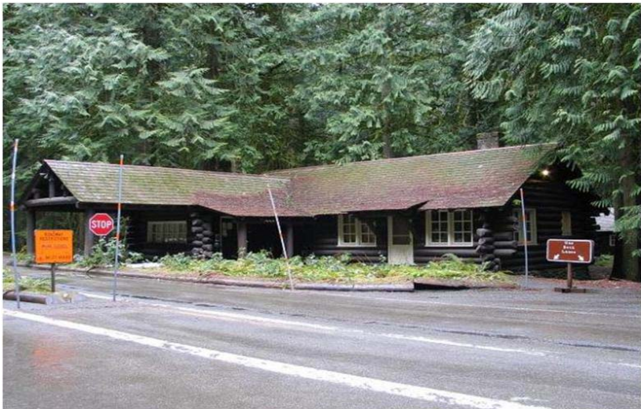
Mount Rainier NP's Historic Nisqually Ranger Station
