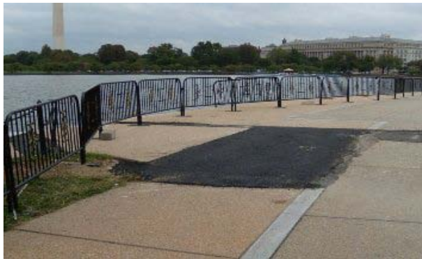
The Thomas Jefferson Memorial's seawall along the Potomac River in Washington, D.C. was sinking into the river's muddy bottom. Interim repairs and barricades protect visitors as the repairs continue.
