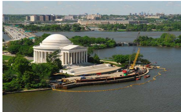
The Thomas Jefferson Memorial's seawall along the Potomac River in Washington, D.C. was sinking into the river's muddy bottom. Interim repairs and barricades protect visitors as the repairs continue.
