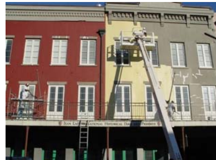
Painting the exterior of the Jean Lafitte NHP headquarters building
