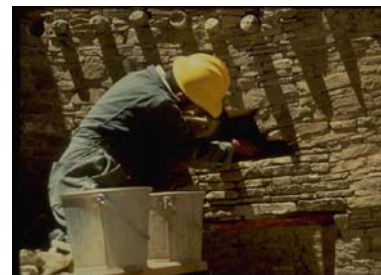
Mason repairs prehistoric stone walls, Chaco Culture NHP.
