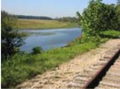
Charles County, Maryland, is planning a new 13.4 mile rail-trail on a former Naval Surface Warfare Center rail corridor received through the FLP in late FY 2006.
