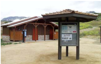
After: New restroom and kiosk were installed with Recreation Fee Demonstration funding and are maintained in "good" condition.
