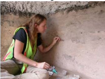
Vanishing Treasures conservator stabilizes interior earthen plaster in rock cut structure, Bandelier NM.
