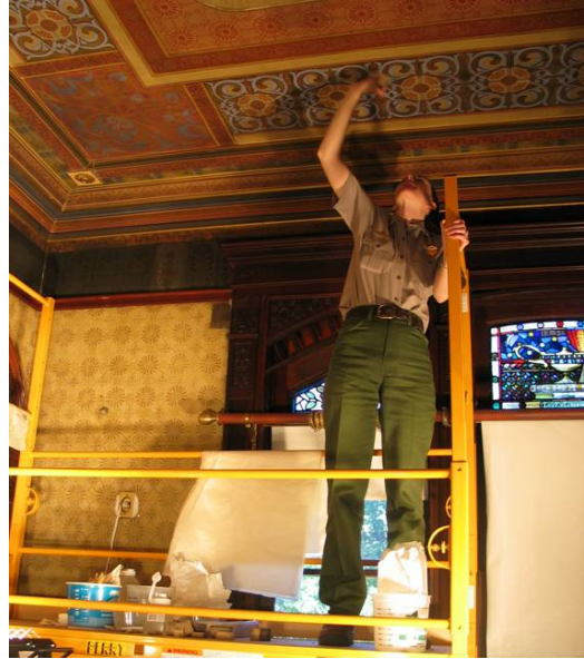
As part of a conservation team, an NPS curator cleans decorated walls and ceilings of the library in Thomas Edison's Home at Edison NHS.
