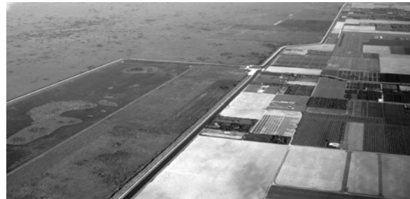
Recently constructed detention areas on the eastern boundary of the park are intended to provide water deliveries with more natural spatial distribution and time while minimizing water quality impacts associated with direct structural discharges. The detention area in this image is the dark rectangle at the bottom left.
