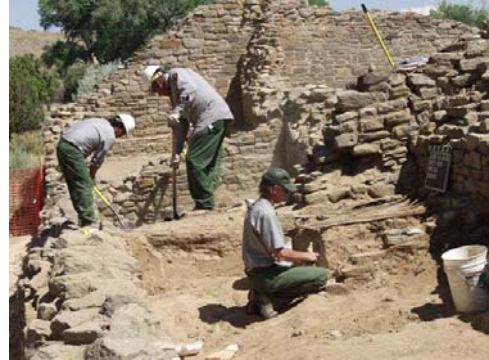
Preservation crew at Aztec Ruins NM removes backfill to install drainage systems and other improvements.
