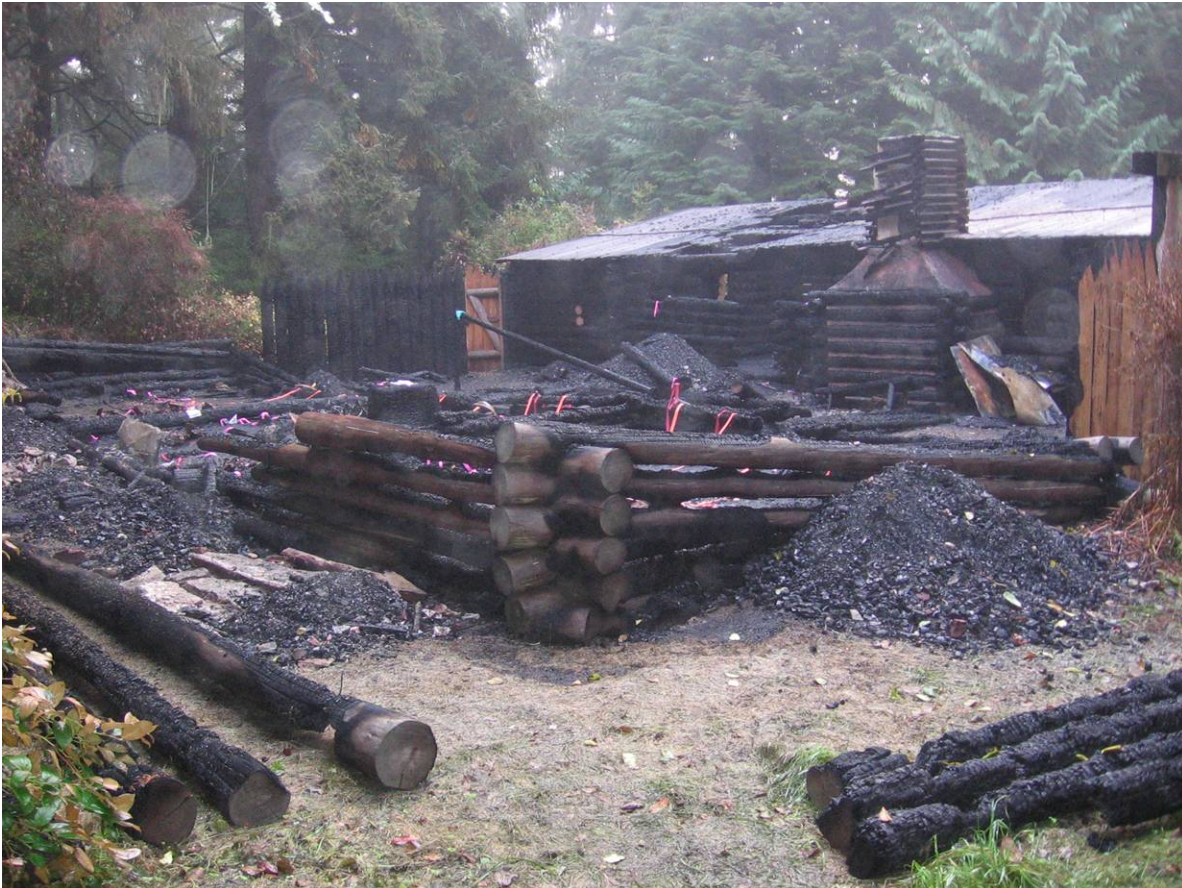
In early October 2005, two months prior to the bicentennial commemoration of the arrival of Lewis and Clark, the 50-year old reconstructed Fort Clatsop at Lewis and Clark NHP is destroyed by fire.
