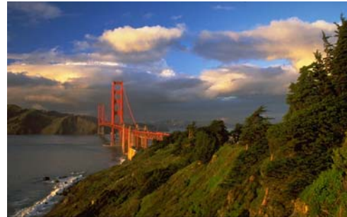
Maintenance operations at Golden Gate NRA are diverse.
