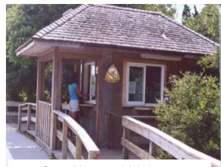
Cape Hatteras Lighthouse Entrance Station
