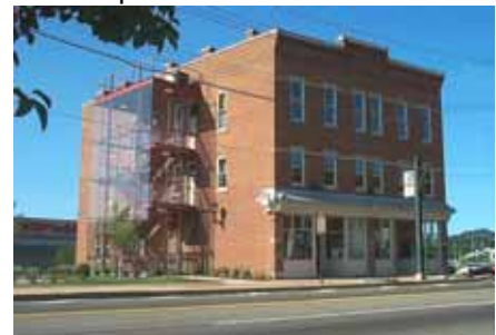
The newly restored 1892 Bost Building now houses the offices of the Steel Industry Heritage Corporation
